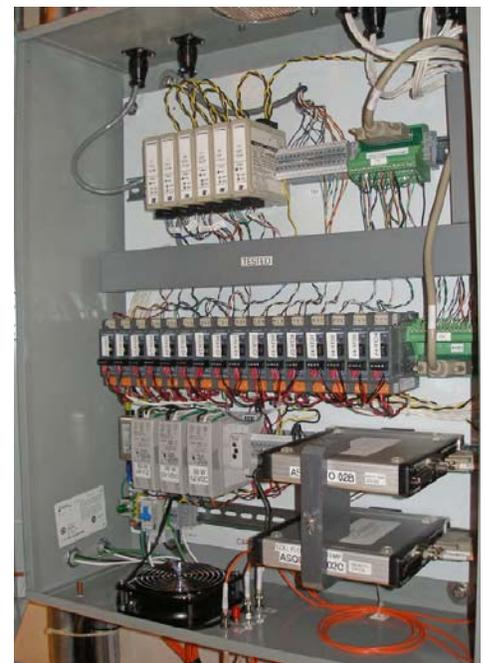
Figure 23. The analog interface box, Box 4, contains two ASQUIRT02 units to echo water cooling information to both PLC and TPS.
