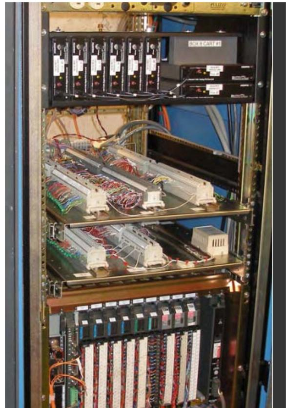
*....but with considerable wiring overhead, shown on the two trays between the Box 8 rack and the PLC.*
